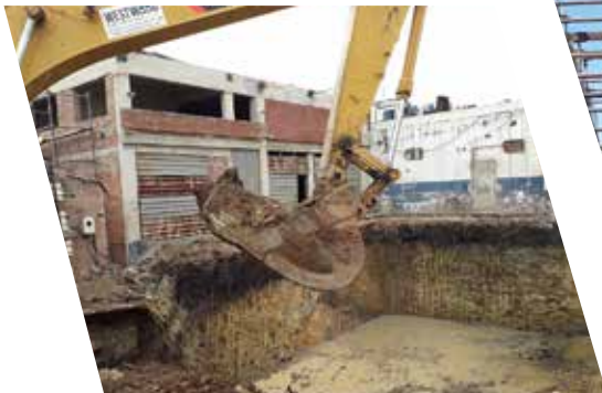
New Shell Service Centre and Fueling Station
